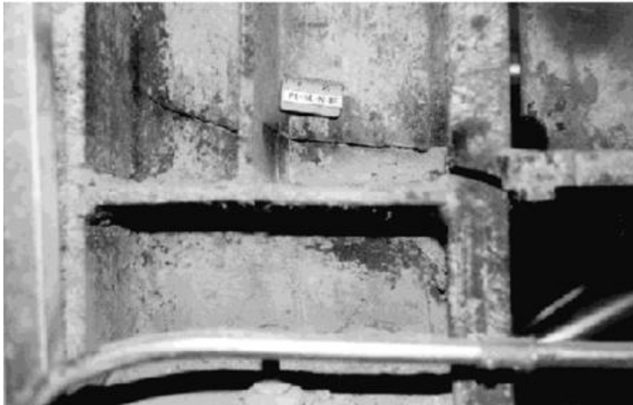
Figure 6.8. Example of a welded steel connection that fractured in the 1994 Northridge Earthquake. Notice that the weld between the flanges experienced a tensile crack that extended across the web of the steel column. Prior to this earthquake, it was generally believed that mild structural steel would ductily bend, but that it would never fracture. .
