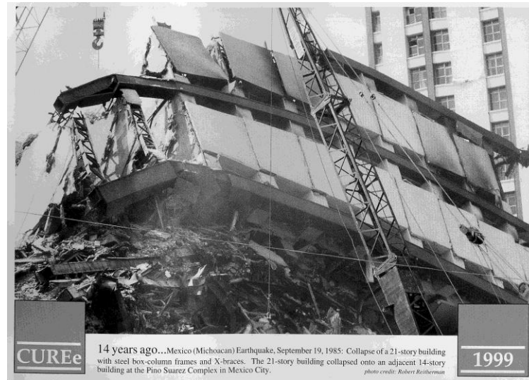
Figure 6.46. Close-up of the left tower in Figure 6.45. Although the three towers were designed to be the same, their behavior was quite different, despite their close proximity to each other. The tower on the right suffered no apparent damage as a result of the shaking. The tower on the left collapsed, while the tower in the middle had a permanent roof drift of about 1 meter. It would be very difficult to explain this difference by current state of the art in numerical modeling of these buildings.
