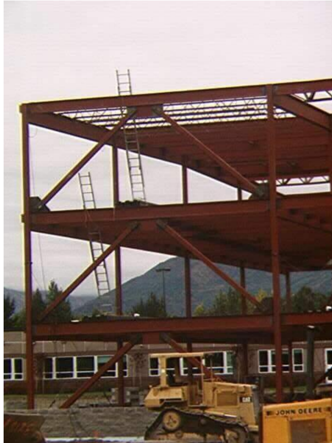
Figure 6.19. Example of a braced steel-frame.
