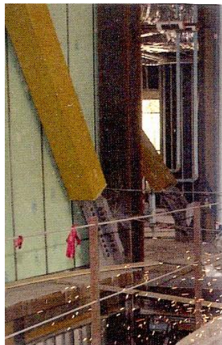
Unbonded Brace in the Broad Center
