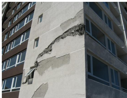
Figure 6.78. Shear failure in a new 25-story shear wall building in Santiago during the 2010 Maule earthquake.
